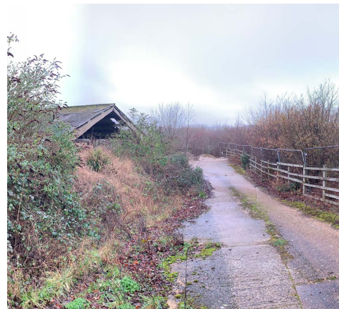
Patcham Court Farm, Brighton
